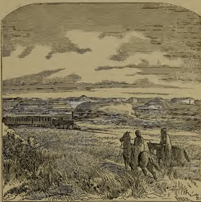
INDIANS VIEWING A TRAIN OF CARS ON THE CENTRAL PACIFIC RAILROAD.
